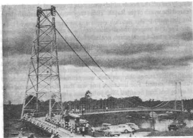
The Satok Suspension Bridge.
